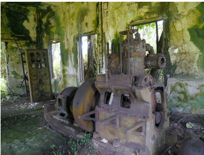
Photo 5. An electric generator used by the Japanese army to power the telegraph during the Second World War.
