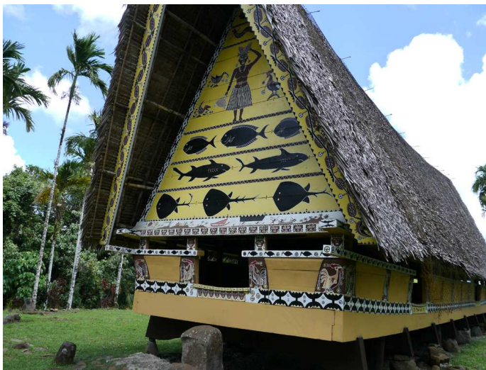
Photo 2. An example of a Bai (Abai) in Aimeliik State. The structure is built on a stone foundation without the use of nails or screws. The outer walls and interior beams are decorated with numerous images.
