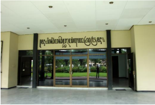
Building of Pubic Water Company.
