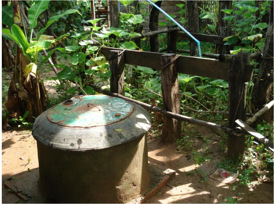
Biodigester: It changes dung into energy for cooking and the lamp
