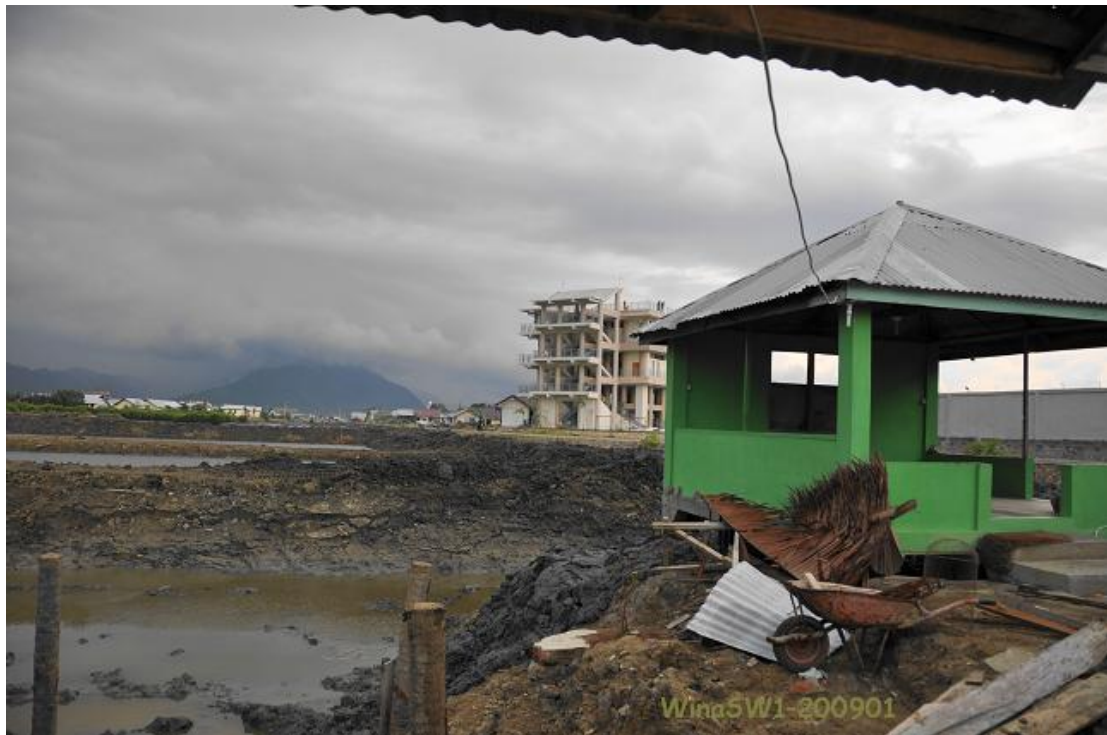
Pic 6. Tsunami disaster escape building made by Japanese in Meuraxa District
